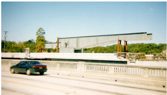
Figure 1 Trunnion-Hub-Girder (THG) assembly.
