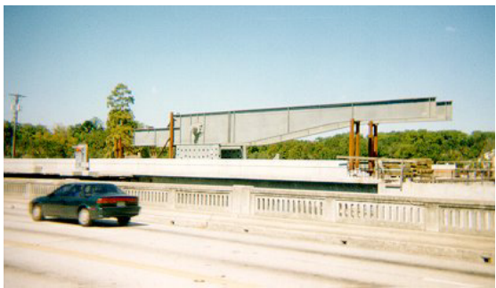
Figure 1 Trunnion-Hub-Girder (THG) assembly.
