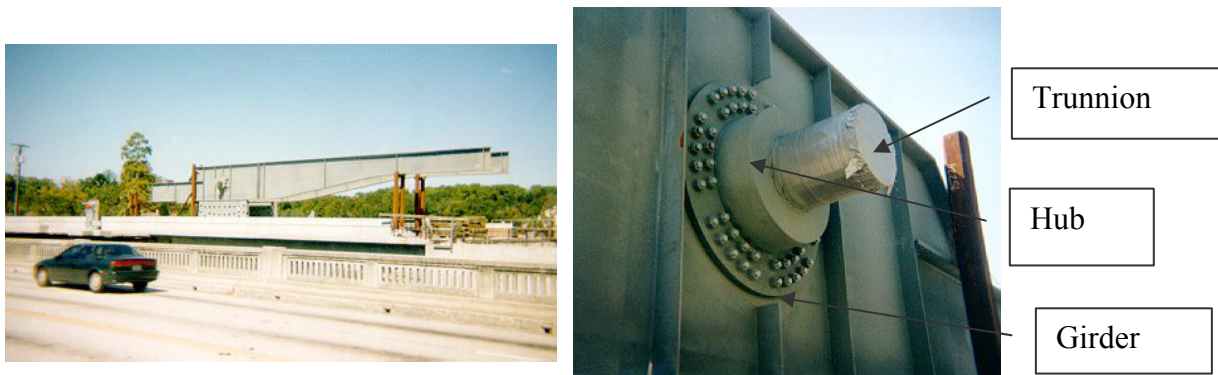
Figure 1 Trunnion-Hub-Girder (THG) assembly.
