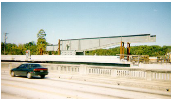
Figure 1 Trunnion-Hub-Girder (THG) assembly.
